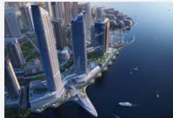
ADDRESS HARBOUR POINT
